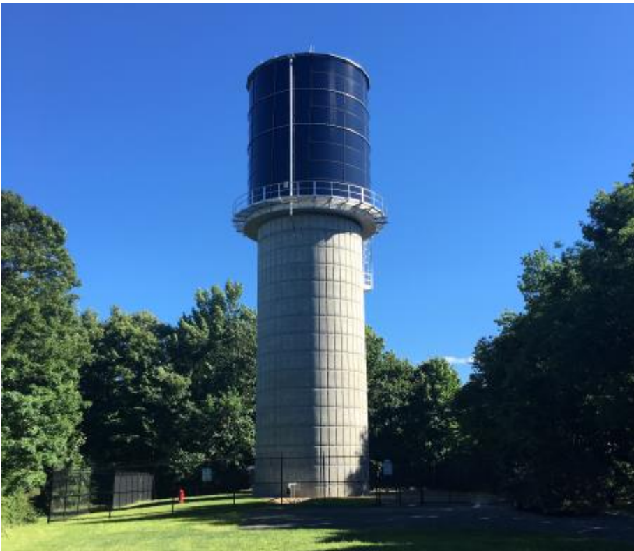
Figure 4 New 210,000-Gallon Elevated Glass-Fused Tank Constructed in 2016
