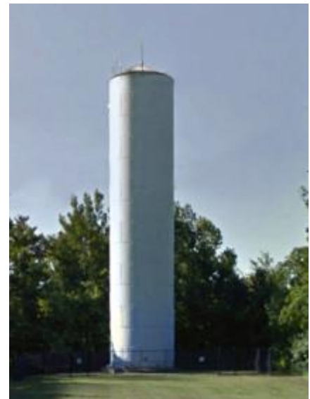
Figure 2 Original Maple Street Tank
