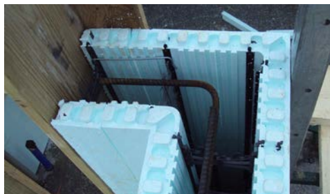
Insulated concrete formed walls
