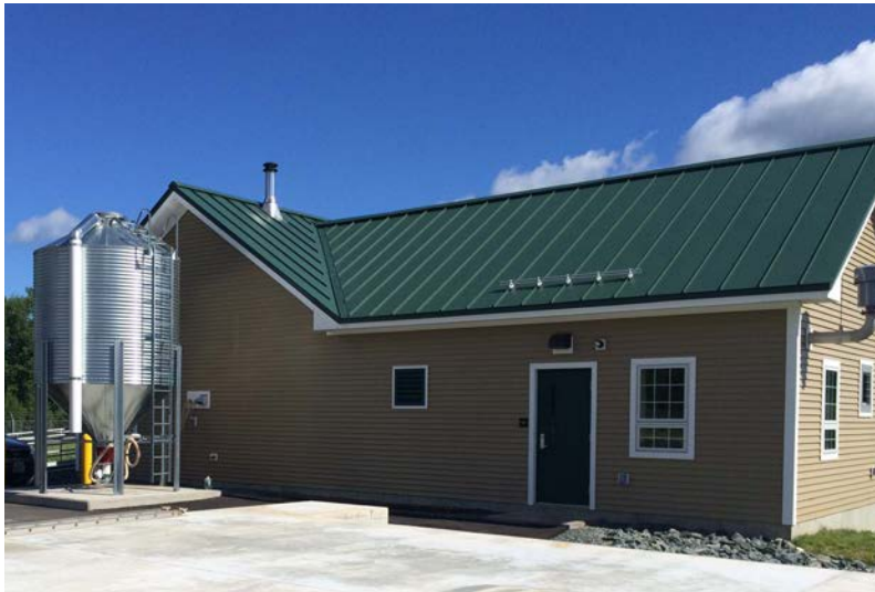
The new Control Building including the wood pellet storage silo
