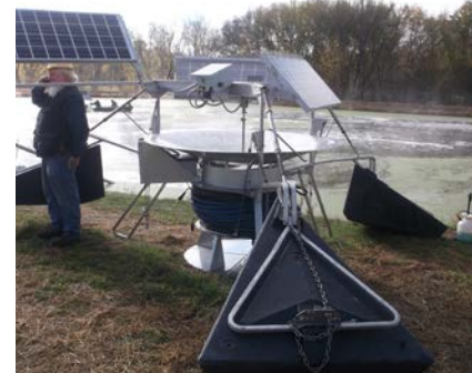
One of the odor-reducing solar-powered floating lagoon mixers
