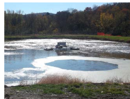
Solar mixer in operation at lagoon
